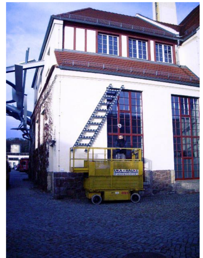
INSTALLATION PROCESS OF THE LADDER: CHERRY PICKER SPONSORED BY UKA+HAUKE
